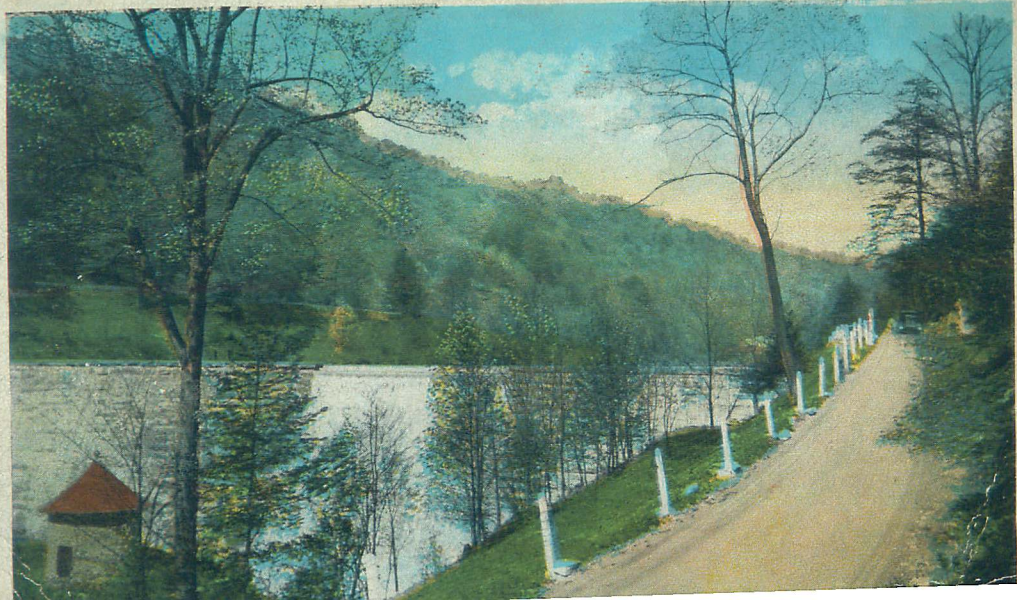
SPILLWAY, ALTOONA RESERVOIR ON WM. PENN HIGHWAY, ALTOONA, PA.
